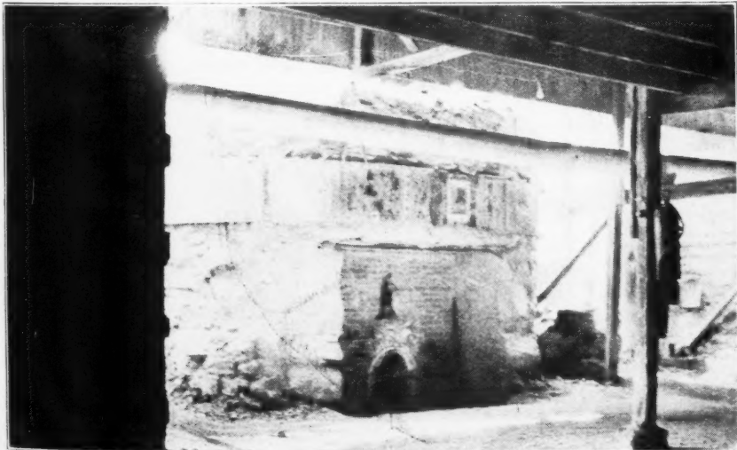
Base of One of the Old Kilns Showing Flue for Forced Draft
